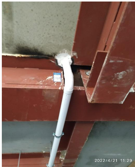
Example of fire stopping in ground floor retail unit
