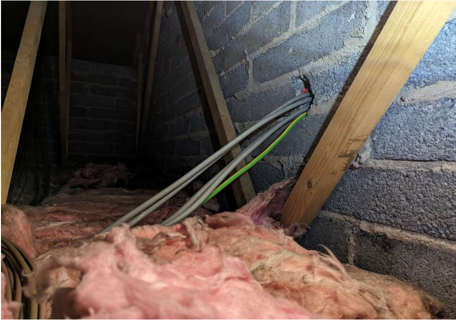
Compartmentation breach in loft of Block 2-7
