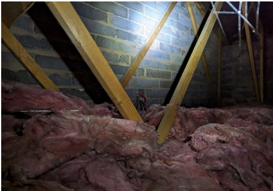
Compartmentation Breach in loft of Block 2-7
