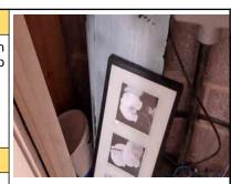
Storage in electrical cupboard: evidence of unauthorised access to a high risk area and potential for build up of combustible items adjacent to electrical equipment.
