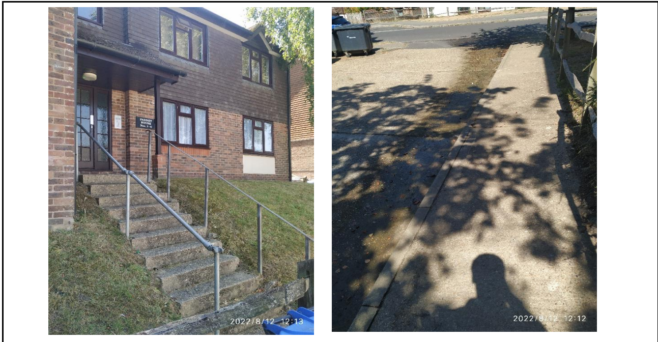
Photo No. 7 Observation: External walkways laid with concrete.
