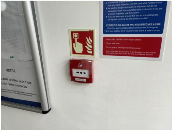
Manual call point(s) in common parts
