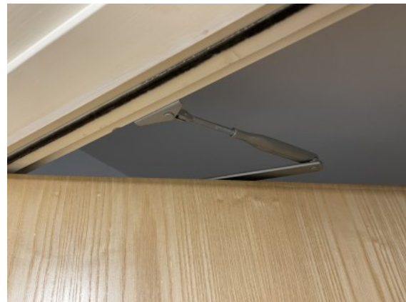
Flat entrance door - Heavy duty self closer
