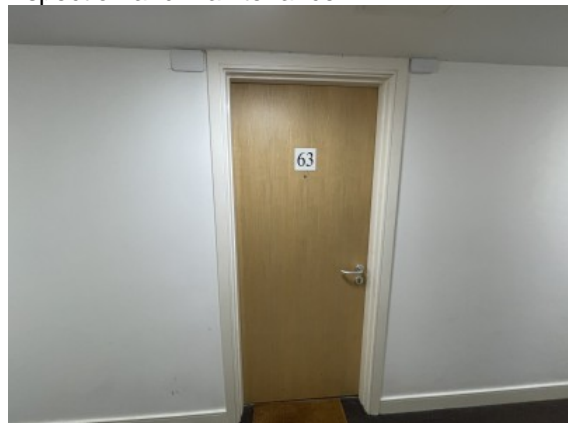
Flat entrance door - Notional FD30S rated assembly
