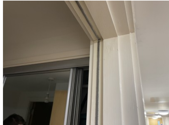
Flat entrance door - Combined intumescent strips/cold smoke seals
