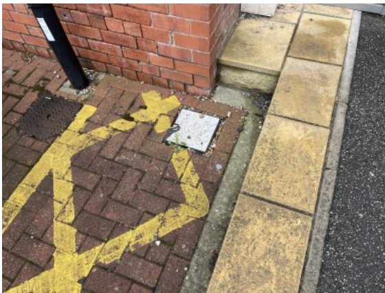
Lightning protection system
