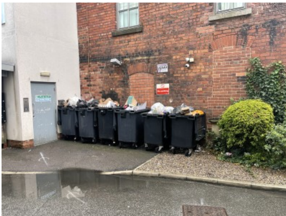
Bins stored immediately adjacent to the rear of the building
