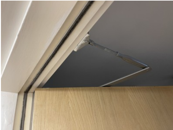
Flat entrance door - Heavy duty self closer
