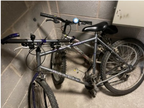
Combustible materials noted in service cupboards
