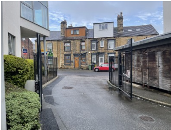
Vehicle entry gates
