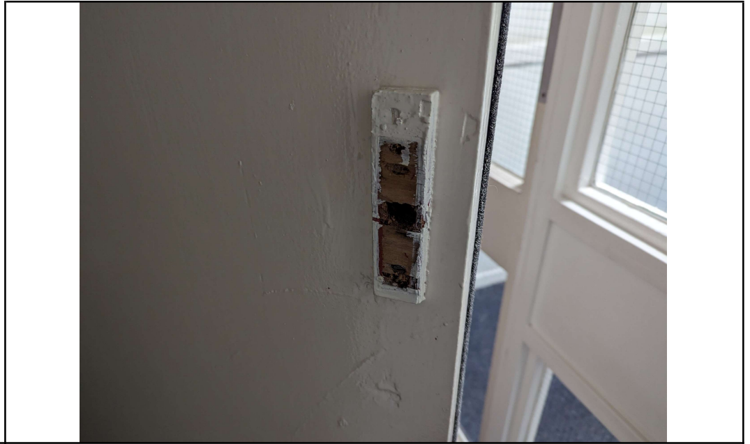
Lock missing from Service cupboard nr 38A/B
