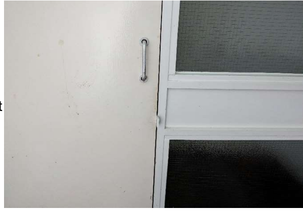
Door gap in excess of 4mm Block 109 GF
