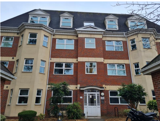
Entrance 4 Front view
