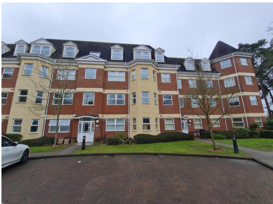
Entrance 12 & 13 Front view
