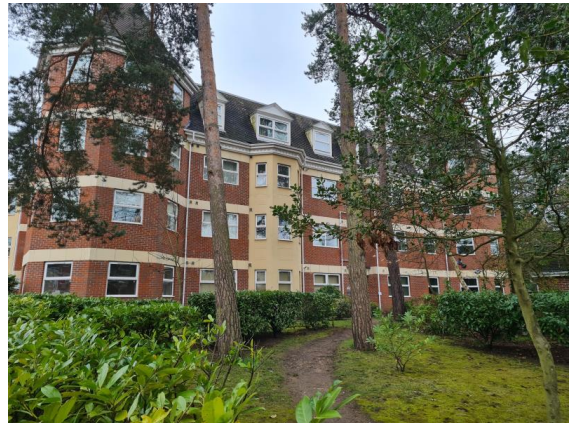
Entrance 15 Front view
