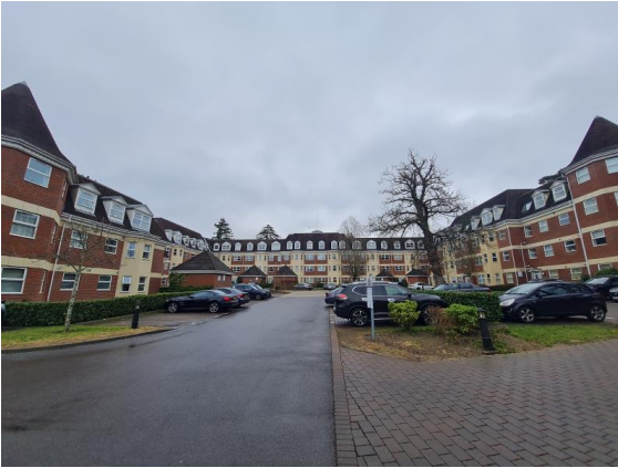
Overall rear view entrances 8-14
