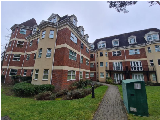
Entrance 16 Front view
