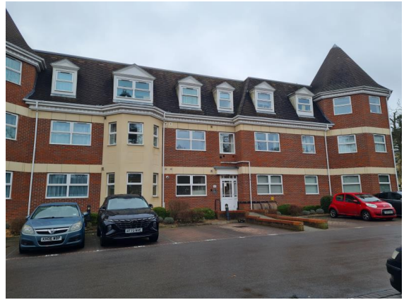
Entrance 7 Front view
