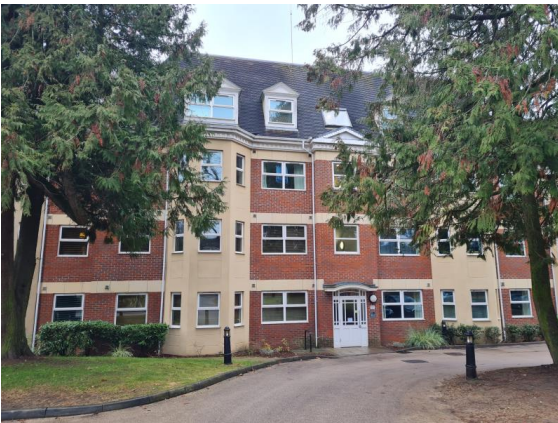
Entrance 2 Front view
