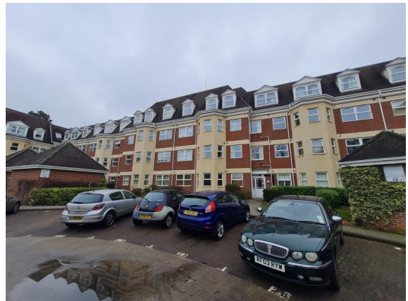
Entrance 10 Front view
