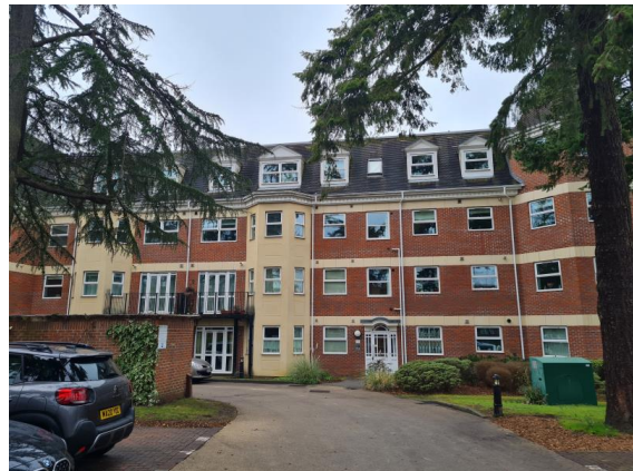
Entrance 3 Front view
