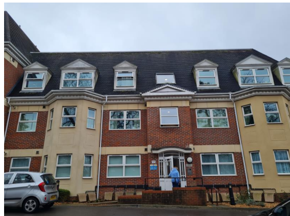
Entrance 5 Front view
