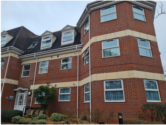
Entrance 6 Front view
