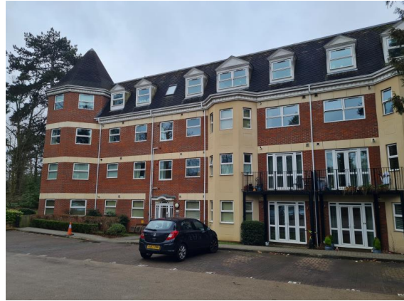
Entrance 1 Front view
