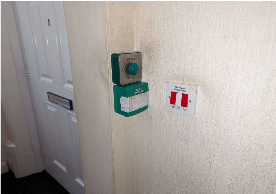
Door Release and Smoke detection tester
