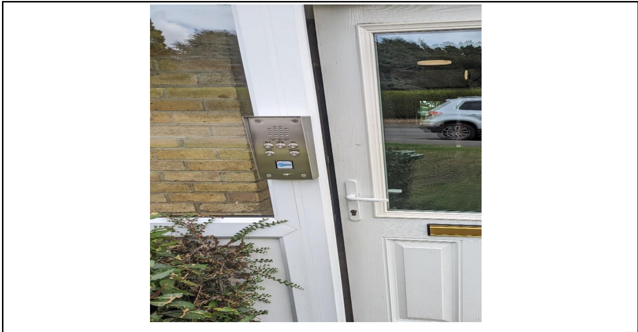
Photo No. 7 Observation - External electronic door entry system in place and manual on exit. Thumb turn exit sign installed during the audit.
