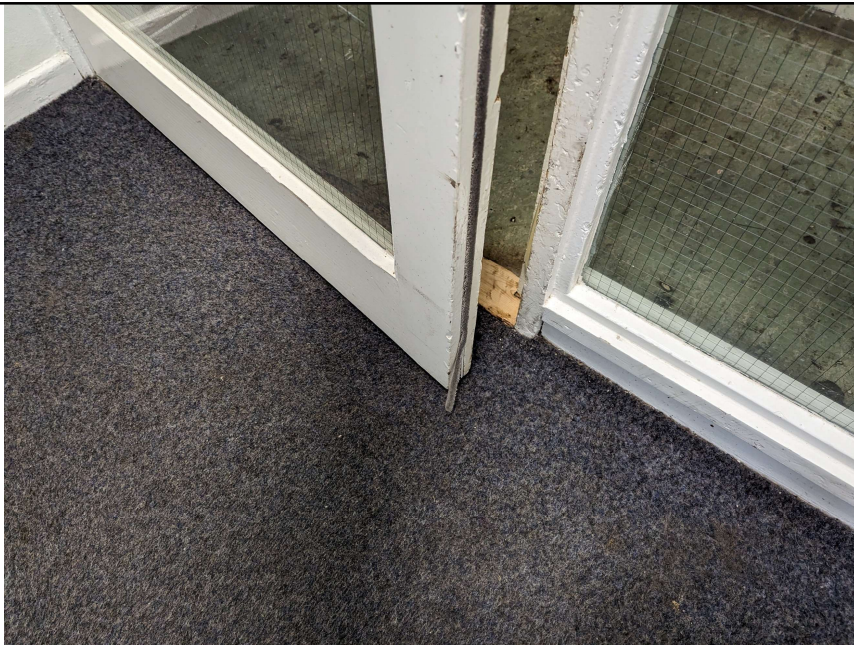
Damaged Smoke seal foyer door in 26 c and d
