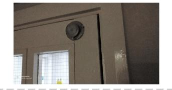
Observation **Referred To** Task ID Priority **Required By:** 31/12/2024 1862641 Both head of stairs communal doors require adjusting Repair - Non **Project Manager** Emergency with to reduce gap to within limits. 2nd floor opposite (Building Safety) flat 24 and leading to flats23 to 34.
