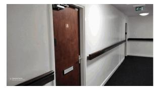
ObservationPriorityReferred ToRequired By:Task IDNew carpets fitted to office door preventing door from self closingInternal - MediumIndependent Living Coordinator14/05/20241813122
