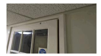
ObservationPriorityReferred ToRequired By:Task IDSeveral breaches were observed in roof spaces and above cross corridor doors.Repair - NonProject Manager31/12/20241886807
